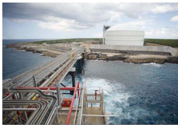
AES Andres Natural Gas Terminal
